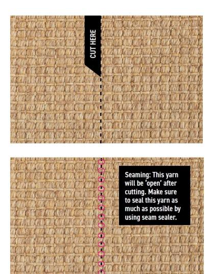
**Figure 1**: Cut 3rd row in from the center seam.
