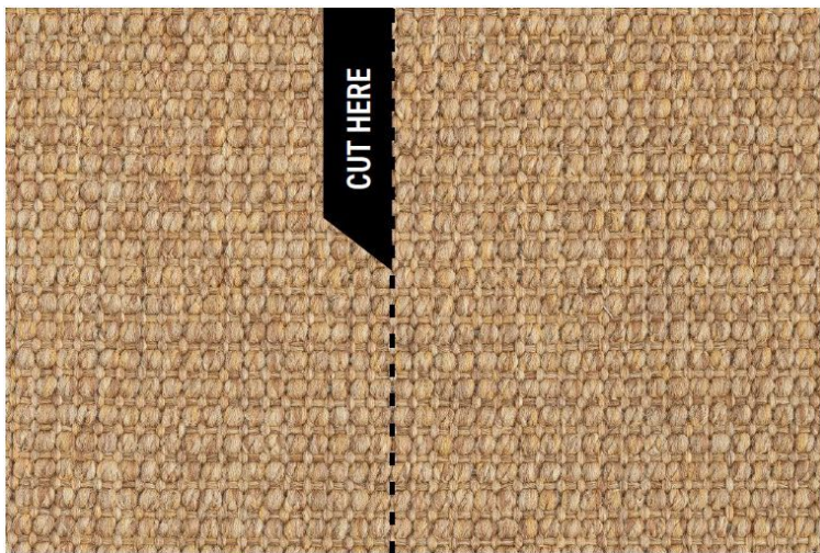
Figure 1: Cut 3rd row in from the center seam. Score first to open the row. Cut with the outside blade.
